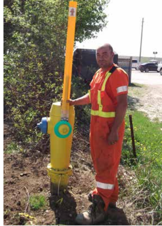
Fire Hydrant Marker
